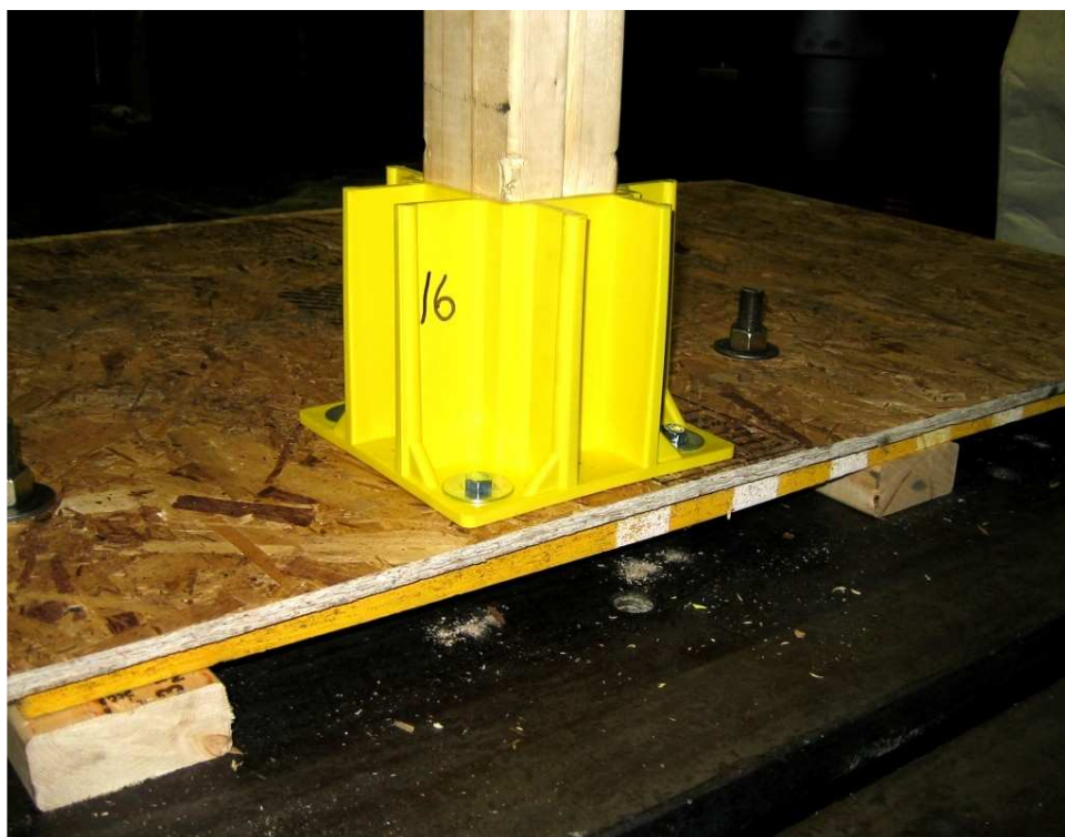
Figure 12: 1-1/8 plywood sub-floor installation
