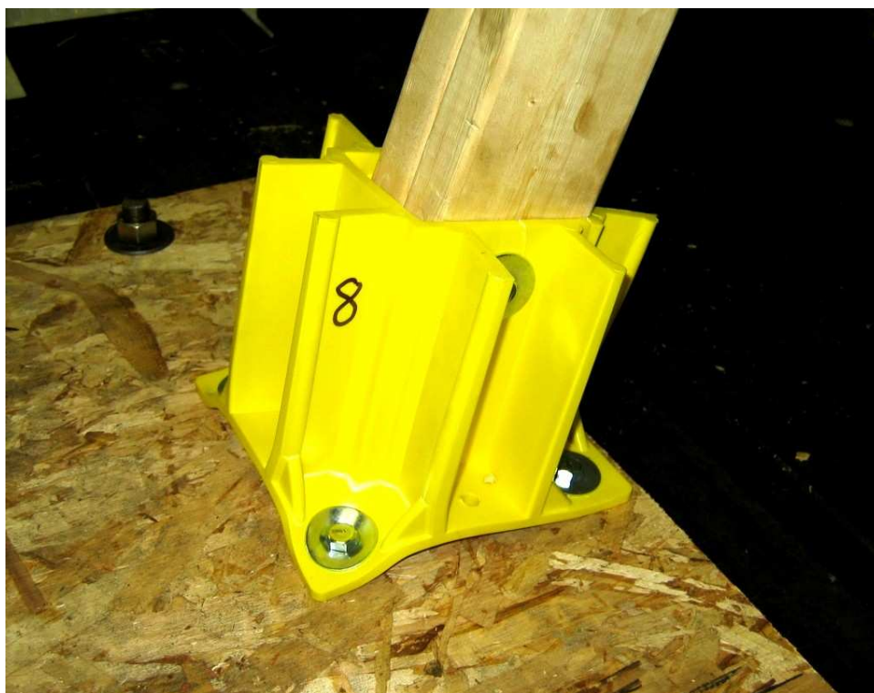
Figure 14: Base deform and crack failures in Test #8
